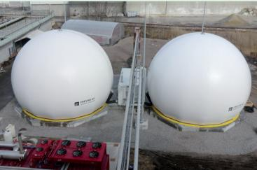
The AAT double membrane gas holder is used as intermediate buffer for the produced biogas, WWTP or landfill gas.
