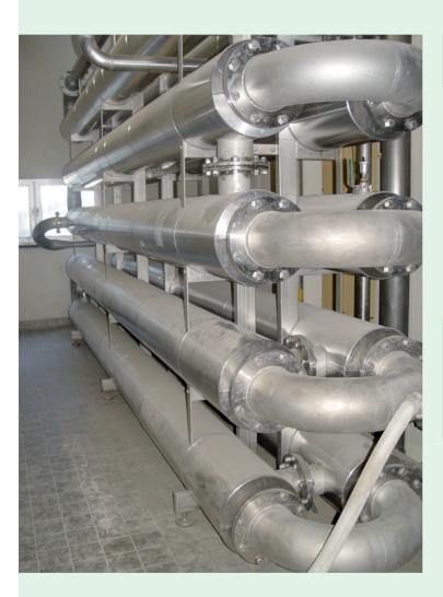
The AAT heat exchanger is used to heat the digested sludge in digester tank.
