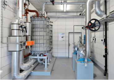
The AAT hygienisation plant is used for (EU conforming) heat treatment of organic waste products which are further processed in biogas plants.
