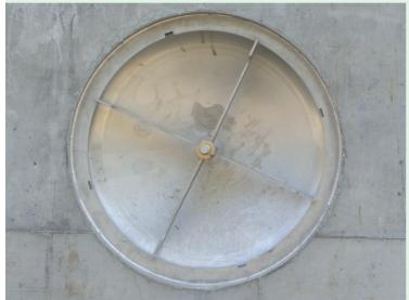
The AAT access opening is used for easy and direct access to the concrete tank for reconstruction or maintenance work.
