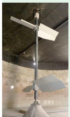
The AAT vertical agitator type VR 15 "Homer" is used for perfect mixing of the substrate in the digester.
