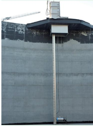
The AAT submersible mixer is used to mix fluids and sludges containing fibres and solids in basins and tanks
