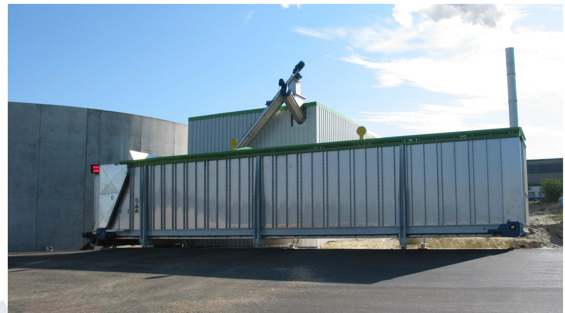
Feeding system with weight-based metering and screw conveyors. Versions in stainless steel
