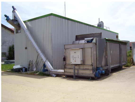
Metering feeder 3 m 3 with collecting, inclined and fermenter screw conveyor.
